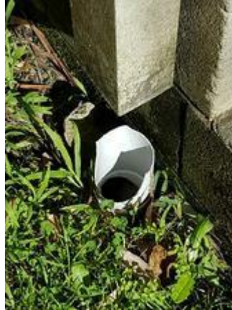
Broken pipes
