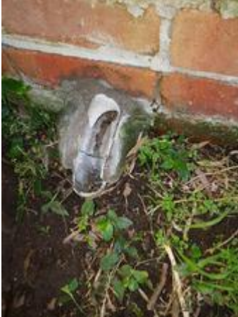
Broken pipes
