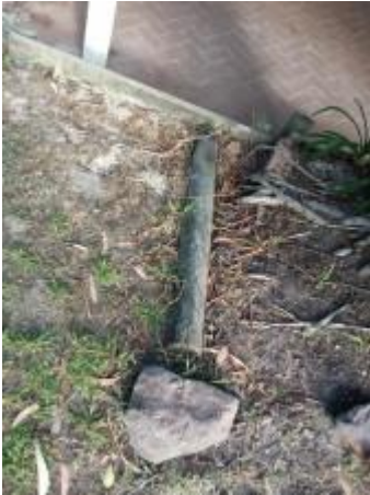
Severe wood rot to electric entry point to main house
