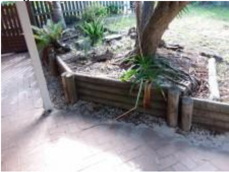
Garden Timbers are in direct contact with the ground and can attract termite activity
