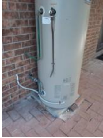
Hot water heater Overflow to the main house and the granny flat a dripping water to external walls this can attract termite activity due to moisture buildup recommend plumbing into drain
