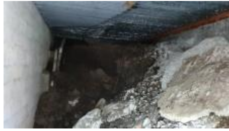
There is evidence of mould in the subfloor areas which may increase in wet weather
