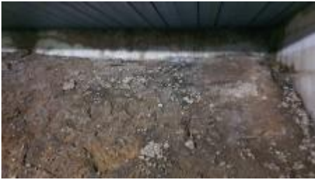
There is evidence of mould in the subfloor areas which may increase in wet weather
